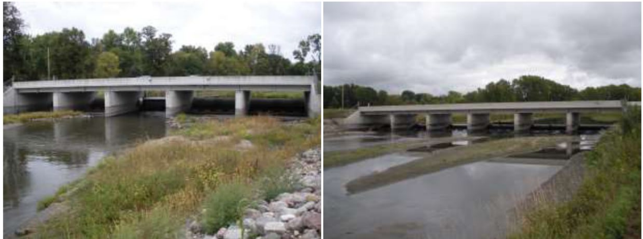
Figure 5. Chippewa Diversion Dam (left) and Watson Sag Weir (right)
