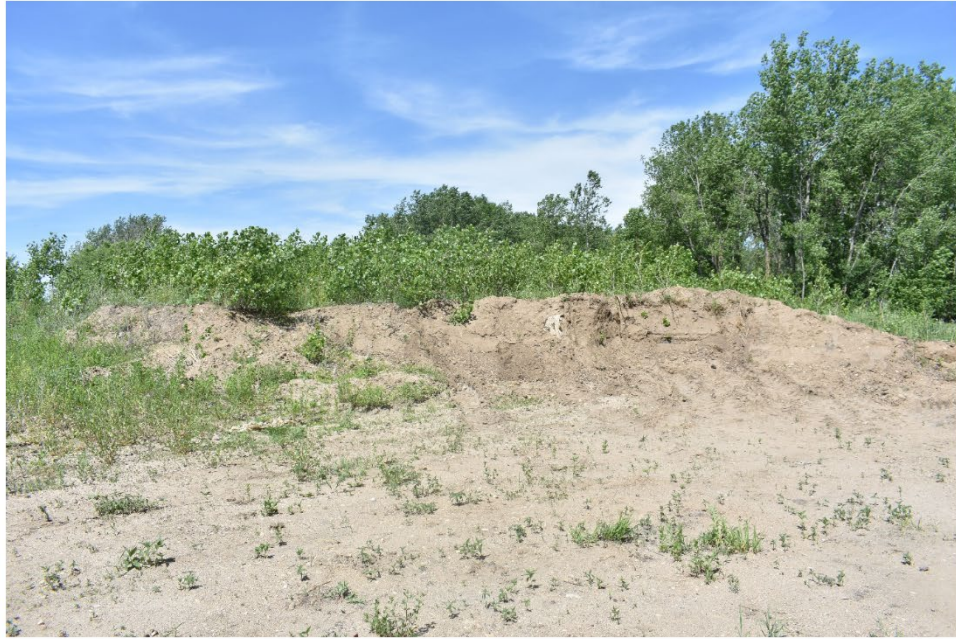
Disposal site 2 – existing spoil pile
