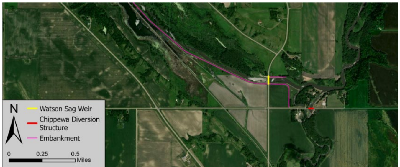
Figure 2. Watson Sag Weir/Chippewa Diversion Dam overview and study area
