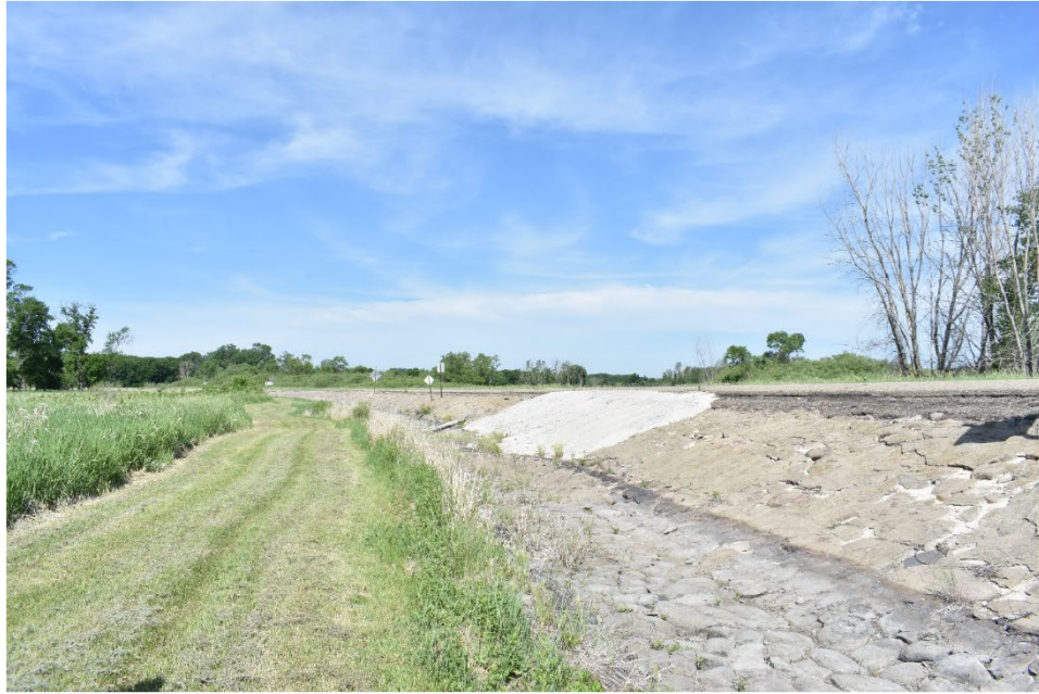
Spillway, looking west
